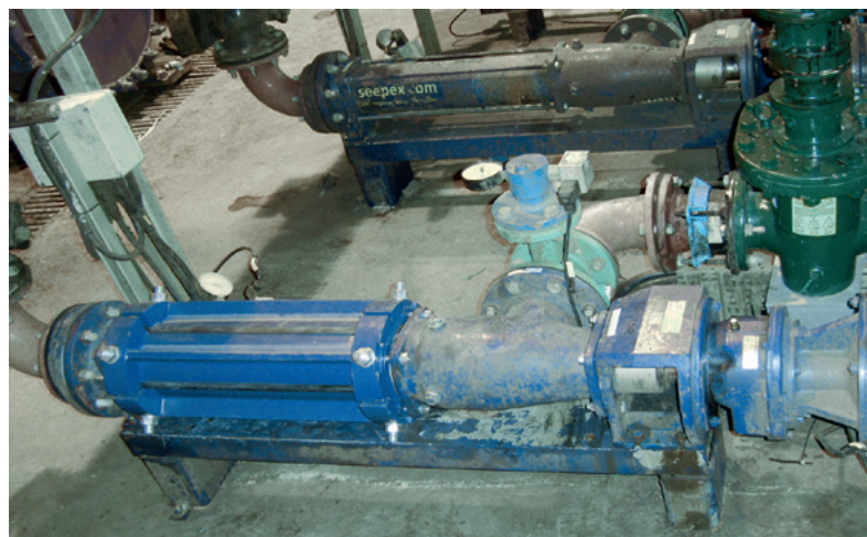
A seepex BN35-6L retrofitted with Smart Stator Technology installed at Osberstown STW
